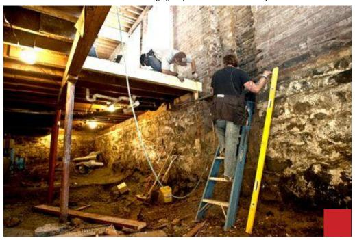
The original mortar and foundation contained local beach sand--seashells and all. Sistered joists against the walls shored up unstable footings.
