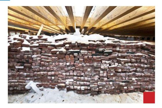
The sorted and stacked bricks are only a fraction of the 28,000 total bricks that workers salvaged for the reconstruction. The original walls were four layers thick, as opposed to one layer for the rebuild, so the tear-down produced thousands more bricks than needed. Neighbors carted off extras to be reused for patios and walkways.
