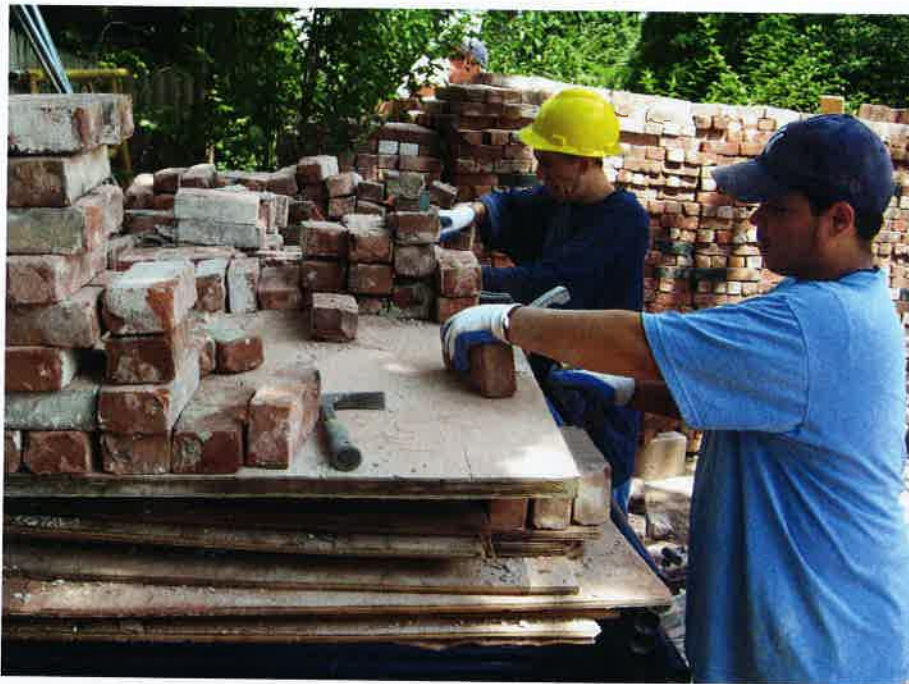
Masons cleaned and sorted thousands of bricks before reconstruction of the exterior walls. “The design intent was to respect the original building,” Jeremy Robertson says. Thus, true double-hung windows in the firehouse all have classic weight-and-chain mechanisms.
