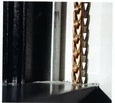
Masons cleaned and sorted thousands of bricks before reconstruction of the exterior walls. “The design intent was to respect the original building,” Jeremy Robertson says. Thus, true double-hung windows in the firehouse all have classic weight-and-chain mechanisms.
